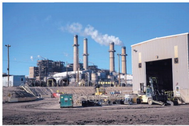
The San Juan Generating Station near Farmington.
